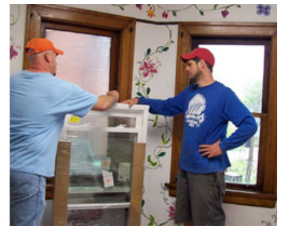
Pat and Kevin work on the windows project.
